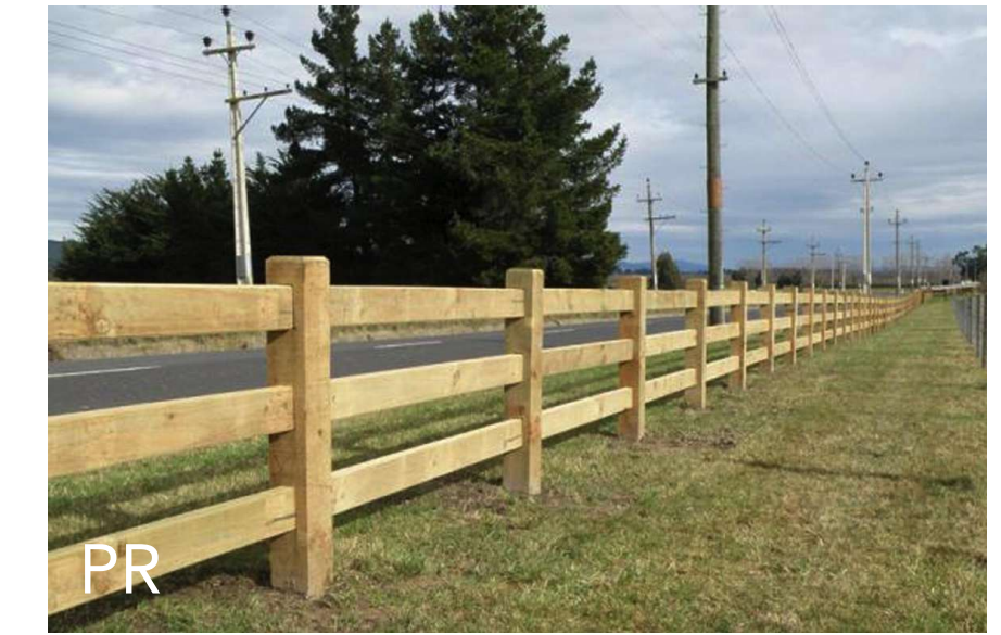
PR Post and rail fence
