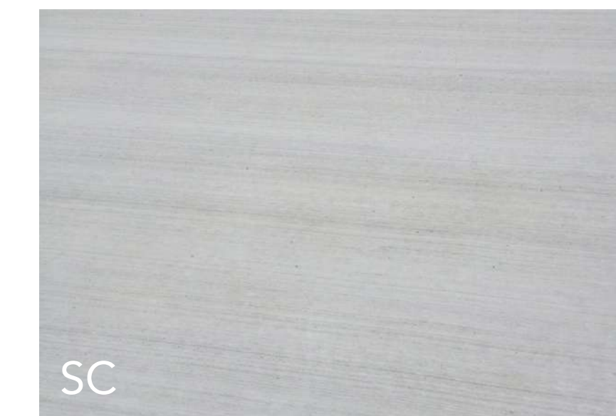
SC Standard concrete, broom finish
