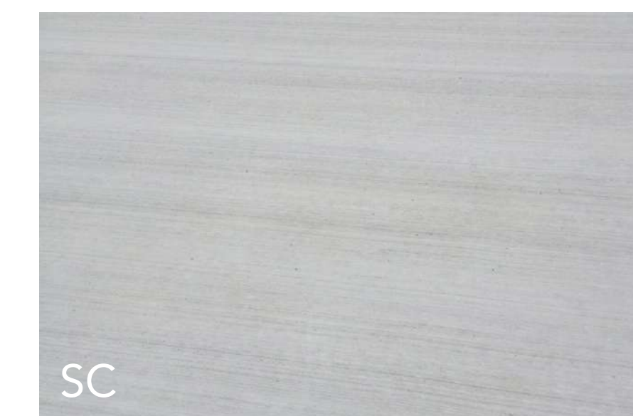
SC Standard concrete, broom finish
